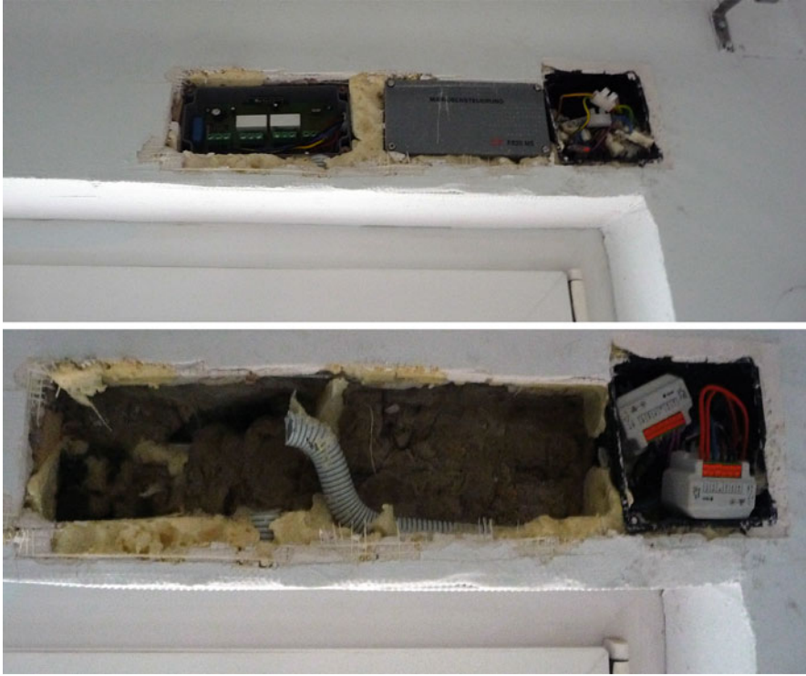
Fig. 7.8 The figure shows the changes in component size between the first installation on the top and the second version on the bottom
