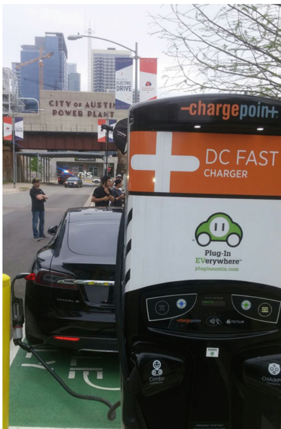
Fig. 7.4 Austin’s “Electric Drive” DCFast dual-standard station
